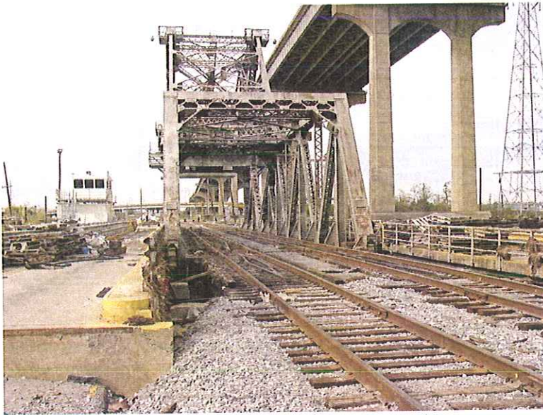
Project E4 – Existing Railroad Bascule Bridge
