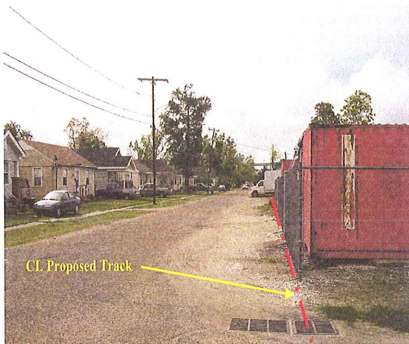
Looking south along St. Joseph Street
