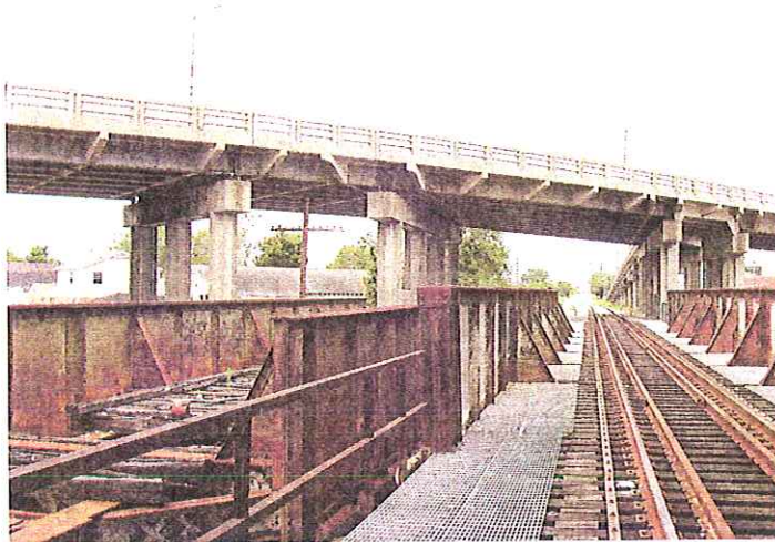
Looking West, Under Palmetto Overpass (Two Steel Plate Girder Rail Bridges)
