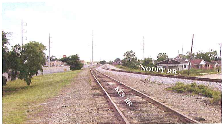
Along Airline Drive Looking East – One Track Would Be Added On The Right Side.
