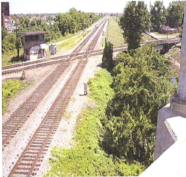
Project E3 – NS Mainline Looking South, Peoples Canal is Right of Track, CSX Mainline Crossing in Center of Photograph
