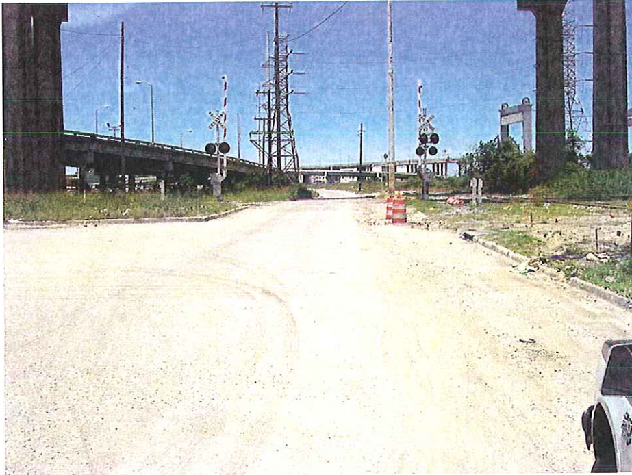
Looking North to Southbound France Road at Almonaster Avenue, Alvar Overpass in Foreground
