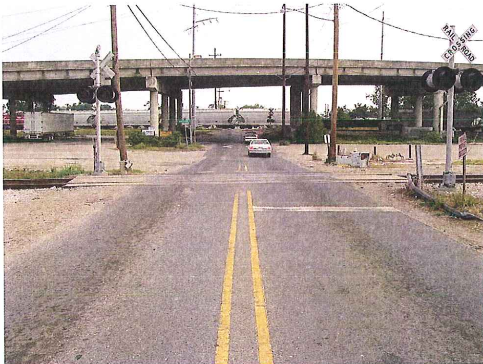
Looking North from Huey P. Long Bridge Leads
