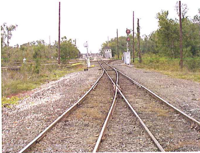
Project W5 – West Bridge Junction from UP Mainline Looking east to HPLB.
