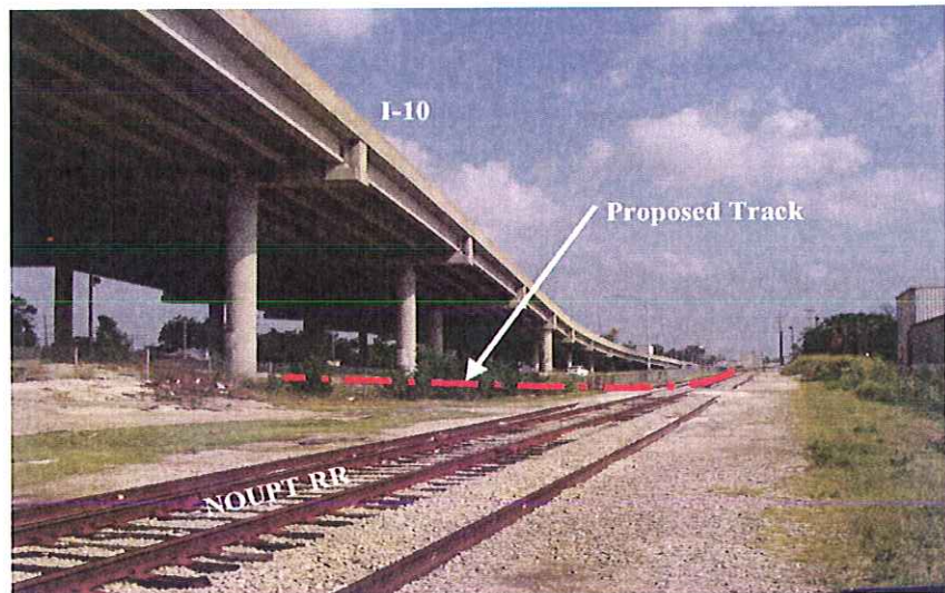
Looking North – East Side I-10/Carrollton Avenue Overpass
