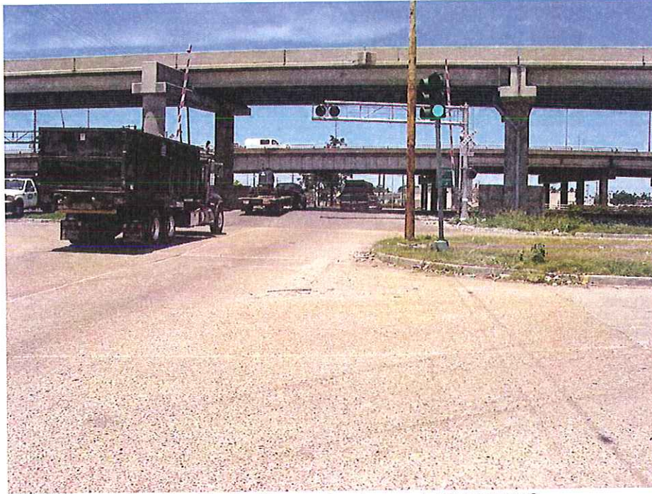
Looking North, Almonaster Avenue in Foreground, Louisa Street/Almonaster Avenue Exist from I-10 above I-10 Main Roadway in Background
