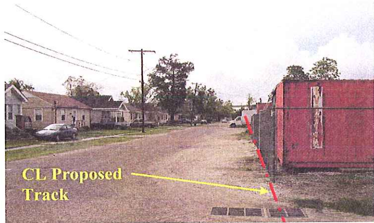
Looking South along St. Joseph Street New Trackage along Right Side of Picture
