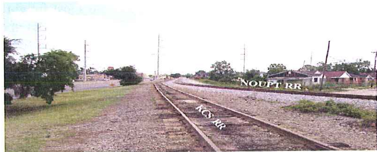
Along Airline Drive Looking East – One Track Would be Added on the Right Side Hollygrove Neighborhood on the Right.
